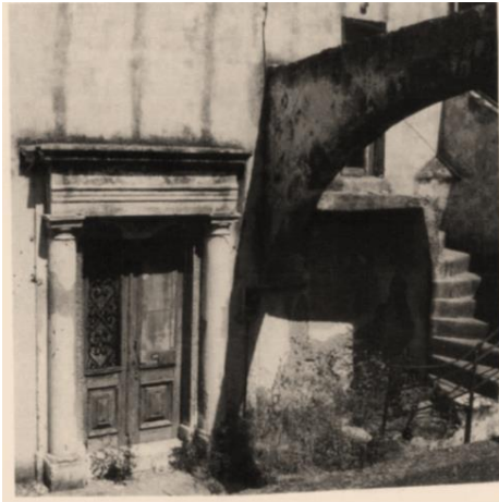
Front entry of the Kahal Tikkun Hazot with a circular stairway leading up to the women's prayer room
